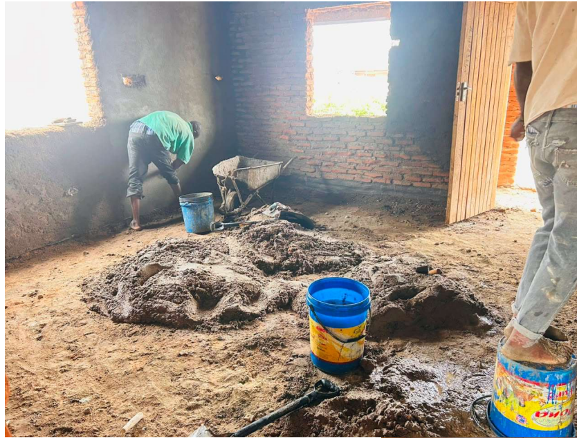
Class room plastering
